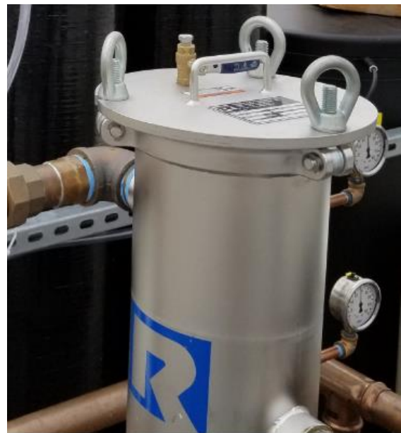
Figure 8. Bag filter housing with hinged wing nut lid
