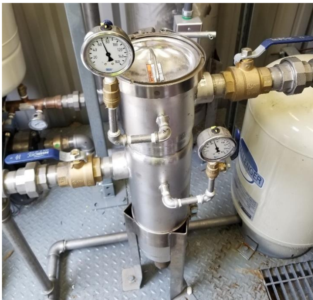
Figure 7. Bag Filter Housing with V-Band Clamp Lid
