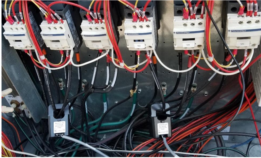
Figure 39. Example of how the CT's should be arranged.
