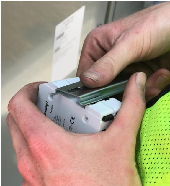
Figure 29. (Above) Mounting fuse block
