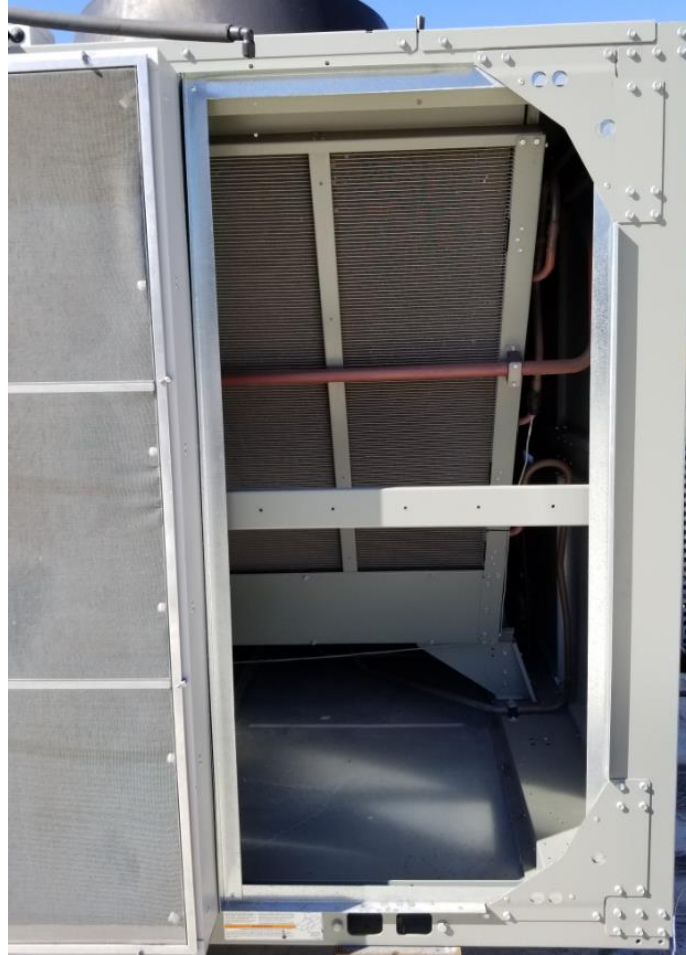
Figure 56. Field Provided Sheet Metal used for mounting EZ-Frames
